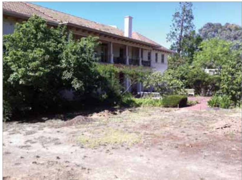
Gardens of Ian Potter House in early 2013, when restoration works began
