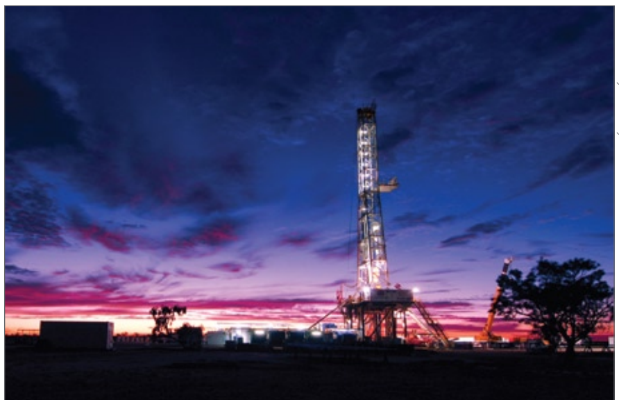
Dawn breaks over a geothermal drilling rig near Innamincka, South Australia
