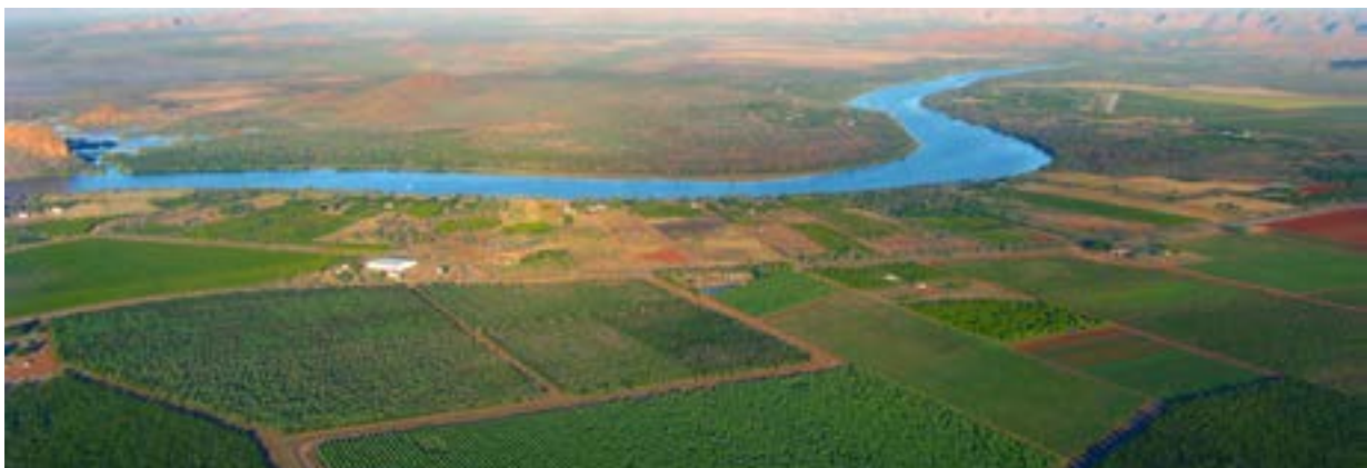
The Ord River Irrigation Scheme, northern Western Australia.
