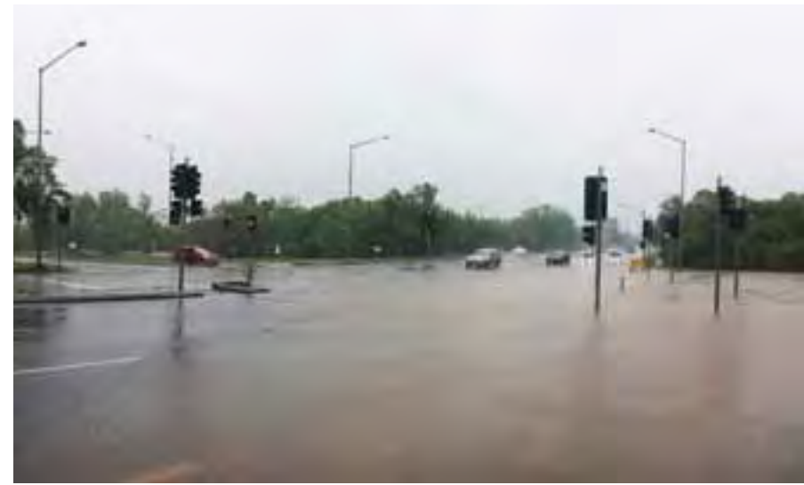
ABOVE: Flooding in Darwin, NT, following tropical cyclone Carlos in 2011. Photo: Charles Strebor
