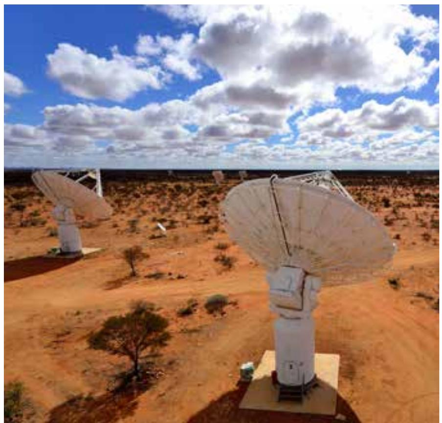
*Precursor telescopes like the South African MeerKAT and HERA, along with the Murchison Widefield Array and CSIRO’s Australian SKA Pathfinder (above) are providing scientists with invaluable knowledge to assist in the design of the SKA’s main telescopes over the coming decade. Photo: CSIRO*
