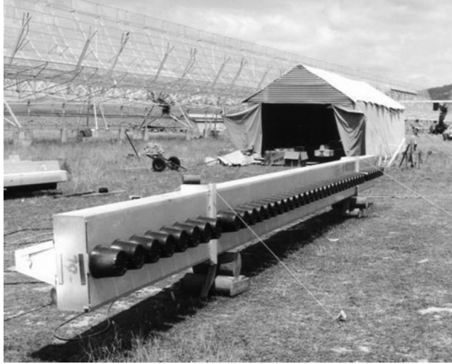
Figure 10. The construction of MOST showing the new feed elements designed to operate at 843 MHz. In the MOST configuration only the east–west arm (visible in the background) of the original cross was used (courtesy of the University of Sydney Archives).
