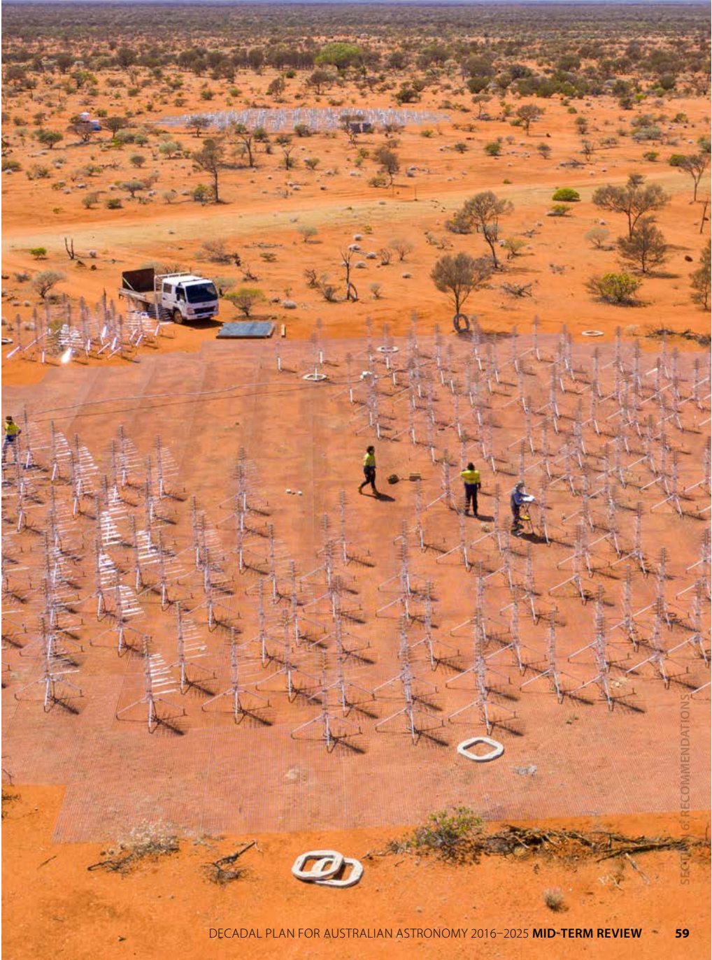
An aerial view of the construction of the Aperture Array Verification System (AAVS) station, a testbed for Square Kilometre Array technology. CREDIT: ICRAR/CURTIN
